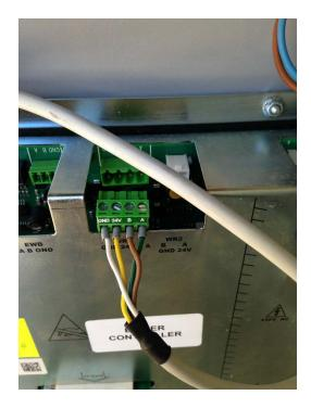
Caution! Wiring should be done when boiler and I/O box are de-energized.
