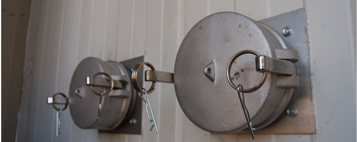
(Photo 3: Installed couplings)
