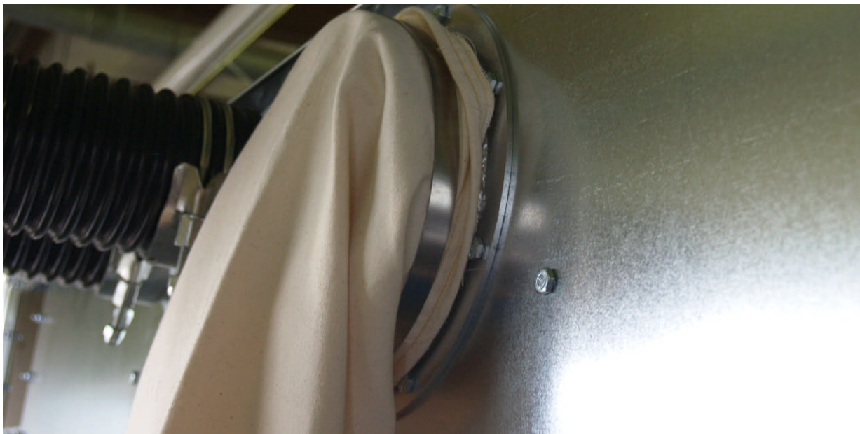
(Photo 7: Installed Filter bag)
